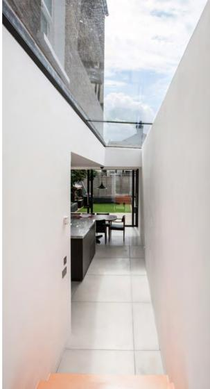
The beauty of the Flushglaze system is its flexibility, for larger areas of glazing the glass panels can be linked together using a variety of different methods.
